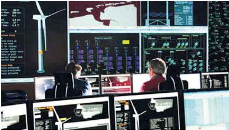
SCADA control center of the offshore wind farm BARD Offshore 1
