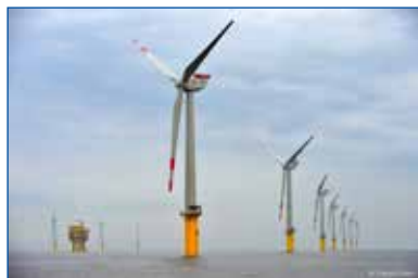
SgurrEnergy completes its construction monitoring role for Borkum
